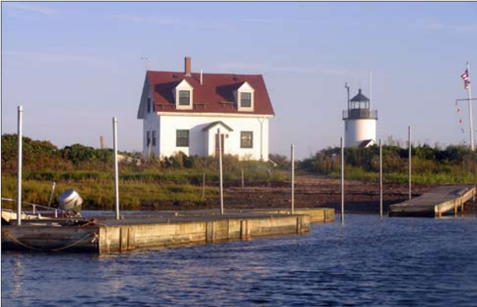
Preparing to install the new floats at Goat Island.
